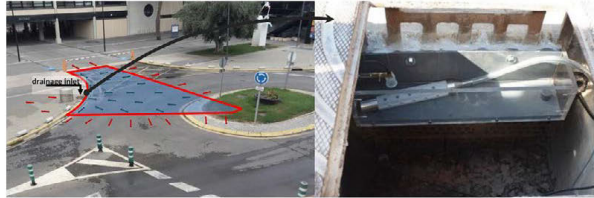
Figure 1. Photographs of the impervious catchment and the sampling chamber (Andrés-Doménech et al. 2018).
