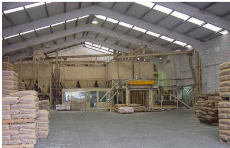
PICTURE 2: General view of a feed mill
