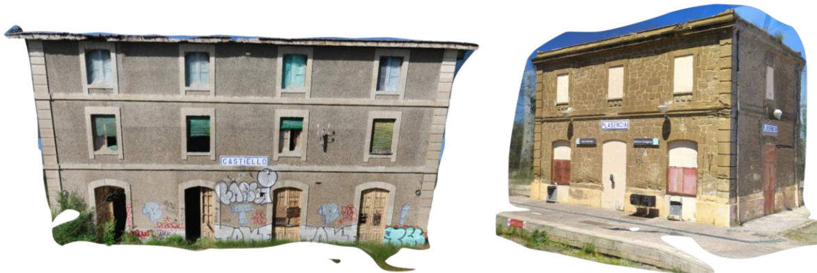
Figures 12 - 13. Point Clouds Obtained through Photogrammetry of the Passenger Buildings at Castiello and Plasencia Stations. Source: Author.
