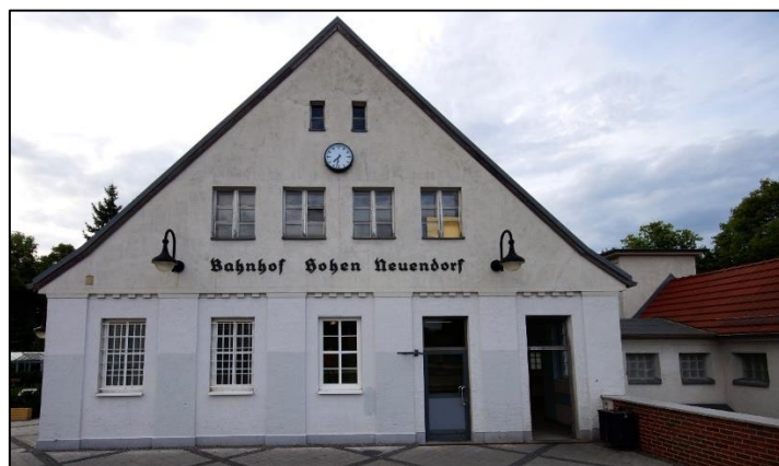
Figure 3: Front view of existent station building (Jivee Blau, 2012)
