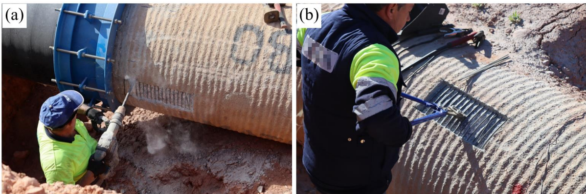
242 Figure 4: Preparation of prestressed concrete pipes. (a) Example of opening a 15 cm high window in one of the 243 prestressed concrete pipes. (b) Wire break with a shear.
