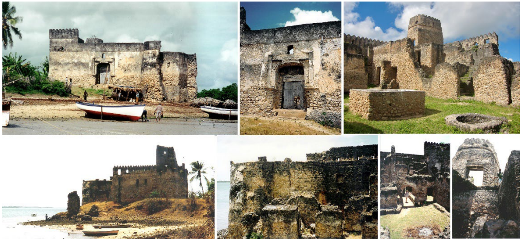
Fig. 7- Several aspects of the condition of the ruins of Kilwa Portuguese-Swahili Fort. (Photos by the Author)
