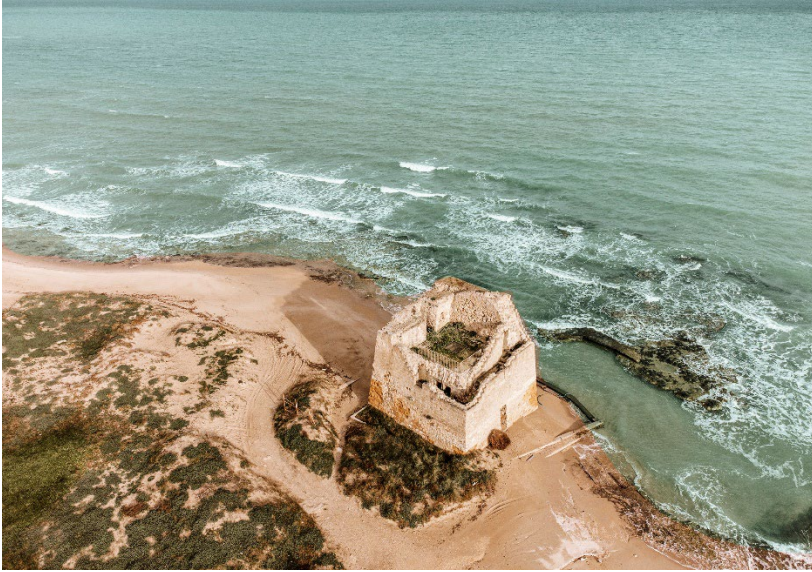
Fig. 5- Aerial view of the tower as it is today (International design competition Reuse the Tower Torre Rinalda (Lecce), Reuse Italy, 2023.)
