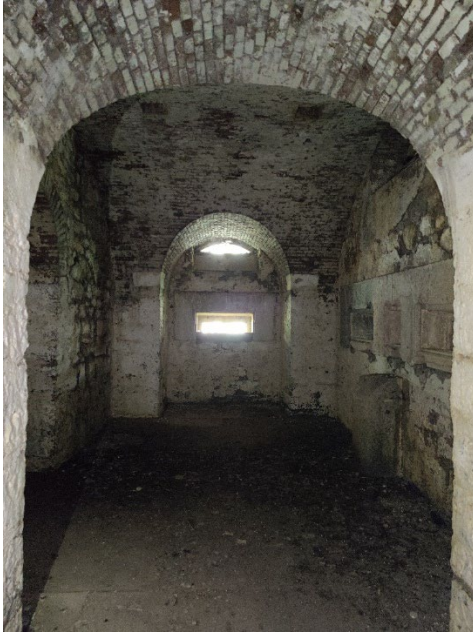
Fig. 10- View of the inside towards the northern side on the ditch (Verdiani, 2023).
