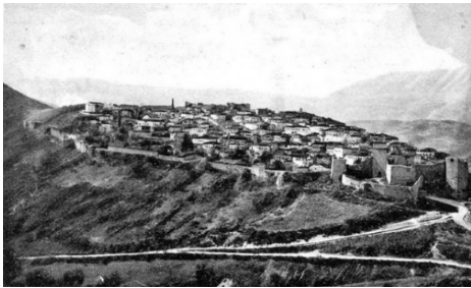
Fig. 7- Photo of the north-western side of the castle of Berat (1960s) showing the hillside free from buildings and vegetation. source: Technical Archive, National Institute for Cultural Heritage
