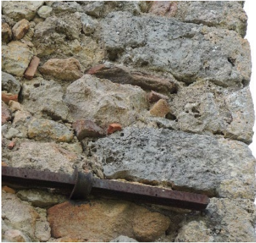
Fig. 11- corner stones made of Cavernous limestone/Breccia di Grotti (photo by A. Arrighetti)
