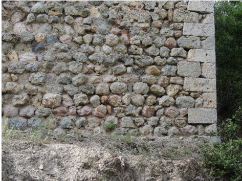
Fig. 6- Detail of the construction technique of Period 2 (photo by F. Fratini)
