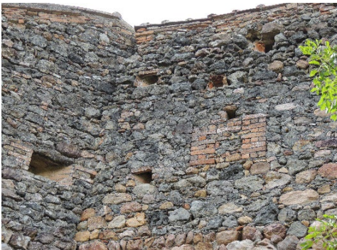
Fig. 12- Detail of the construction technique of Period 4 (photo by F. Fratini)
