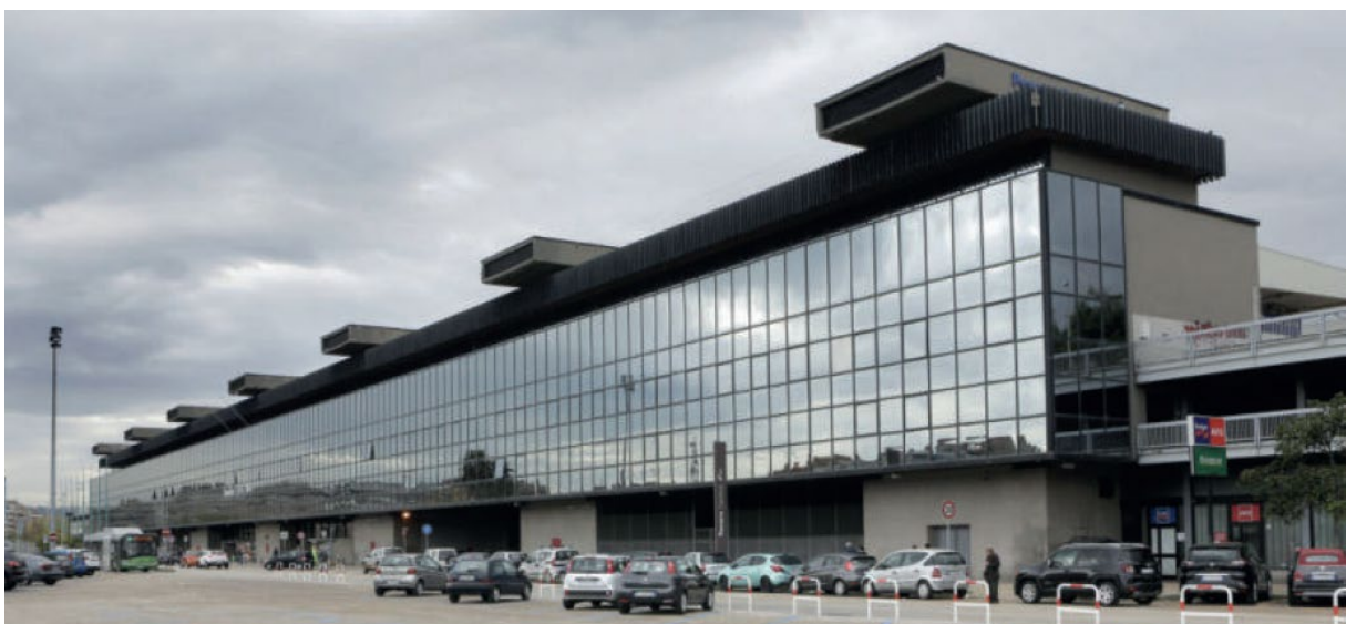
Fig. 5. View of the main façade
