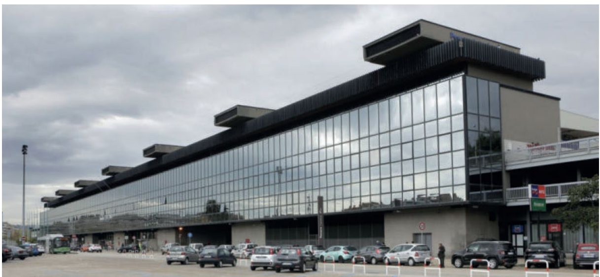
Fig. 5. View of the main façade
