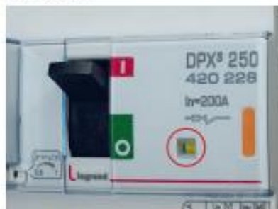
Tripped (Residual current fault)
