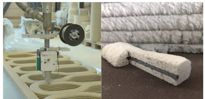
Fig. 9. Extrusion-based printing of concrete reinforced with embedded steel cable (left, courtesy TU Eindhoven) and cross-section of layer reinforcement with carbon fibre (right, courtesy of TU Dresden).
