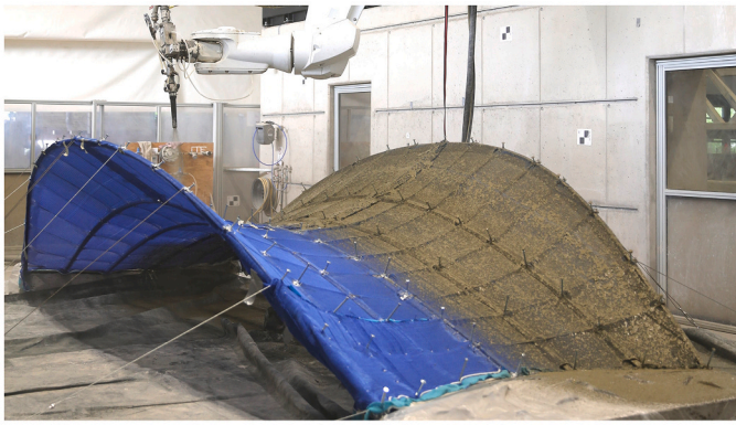
Fig. 18. KnitCrete bridge; application of the first layer of robotically sprayed concrete (left, ©ITE, TU Braunschweig), and the final demonstrator (right, © J. Bergmeister/TUM).
