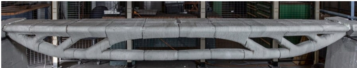
Fig. 23. Topology optimised 3D printed post-tensioned bridge assembled from smaller elements [90].
