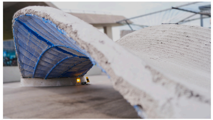
Fig. 18. KnitCrete bridge; application of the first layer of robotically sprayed concrete (left, ©ITE, TU Braunschweig), and the final demonstrator (right, © J. Bergmeister/TUM).
