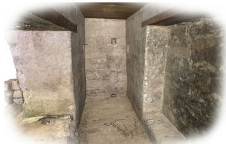
6J2-Sub2 Building + Structure 1 Interior
