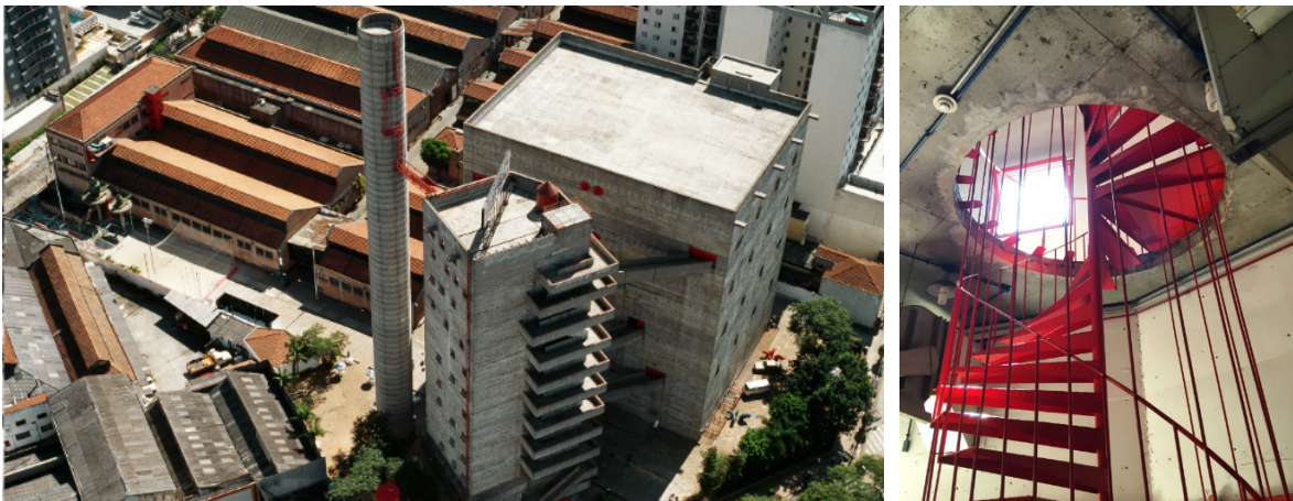
Figure 6. SESC Pompéia (1987-1988) steel staircase.
