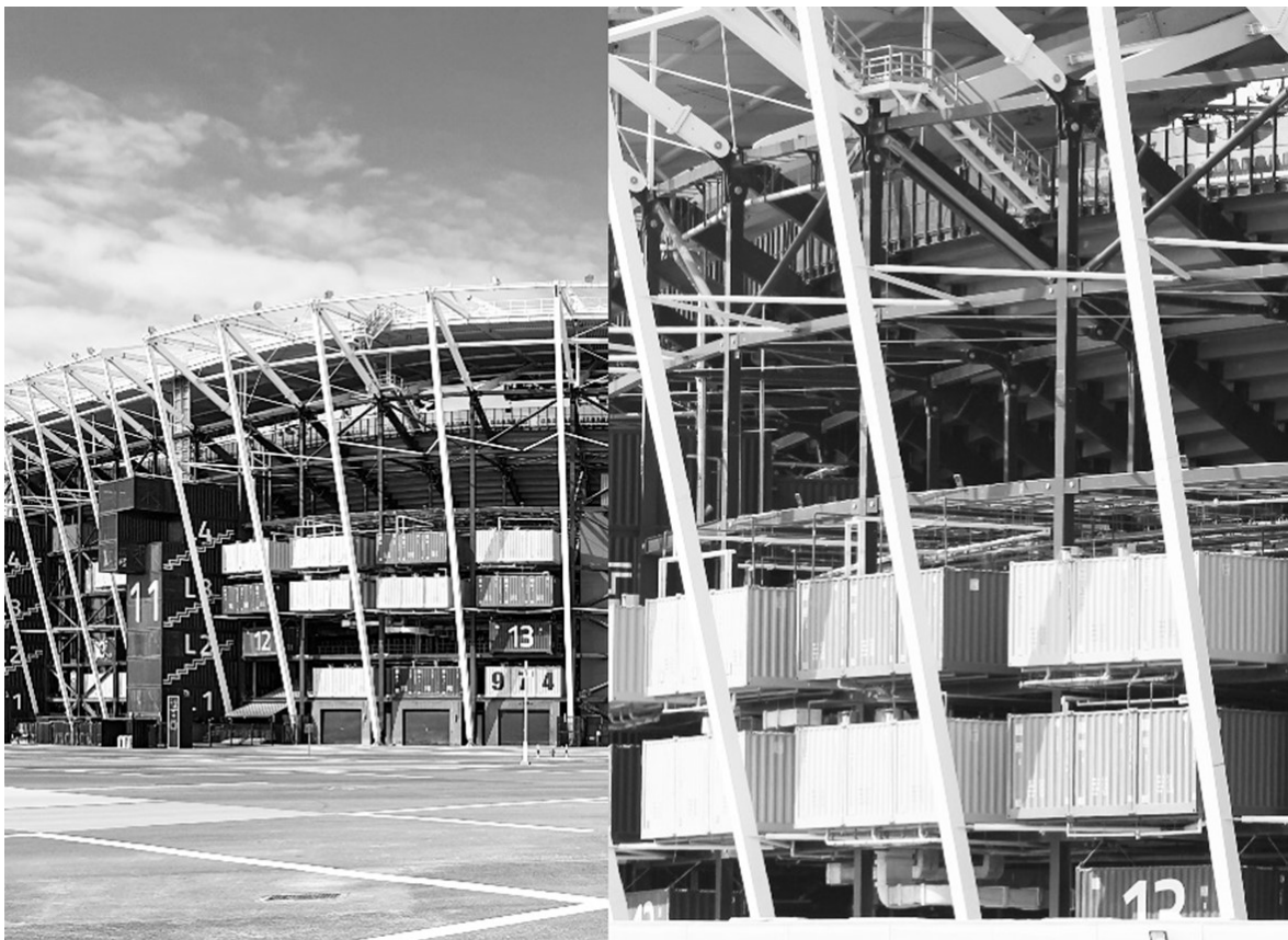
Figure 11. 974-Stadium (Doha, 2021), is the first example of a stadium that can be completely demountable. Built with recycled containers for the Qatar World Cup, it is the symbol of a quite consolidated technological trend for large sporting events to build infrastructures that are partly or completely adaptable, demountable, flexible and resilient (the latest Olympics in Paris are a clear example of this approach).
