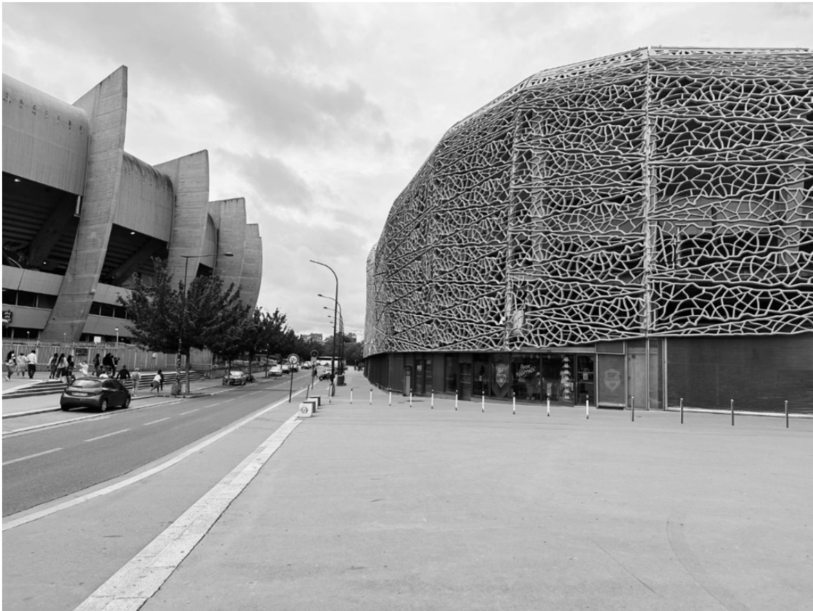
Figure 5. Two stadiums in Paris are a few meters from each other of different generations. On the left the brutalist stadium by Roger Taillibert (1972, Parc des Princes, IV Generation), on the right the rugby stadium (Jean Bouin, 1925, then almost completely rebuilt in 2013, V Generation) with the technologically advanced facade in GRC panels which offers a new aesthetic perception (more of a museum than a stadium) of the large building in relation to the urban context.
