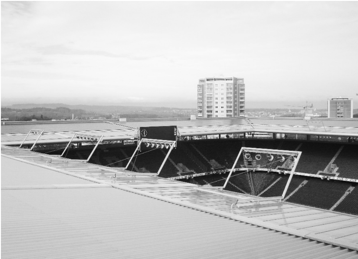
Figure 9. Wankdorf Stadium (Stade de Suisse, Bern, 2005). An urban stadium that until recently was the largest roof-mounted photovoltaic power plant in Europe, it houses public functions such as university spaces.
