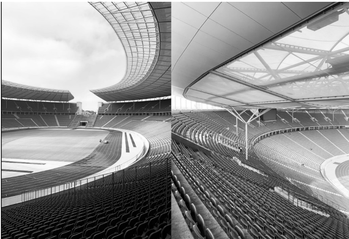
Figure 4. Olympic Stadium (Berlin, 1936 opening, 2006 redevelopment). Example of a regime stadium (II Generation) completely renovated and updated with respect to the requirements for the major competitions of the new millennium (in this case, the 2006 Football World Cup). The approach combined the philological conservation of the old arena with the addition of a new technologically advanced covering from a material (composite textile membranes) and structural point of view and with a strong symbolic impact (lightness versus heaviness of the regime).
