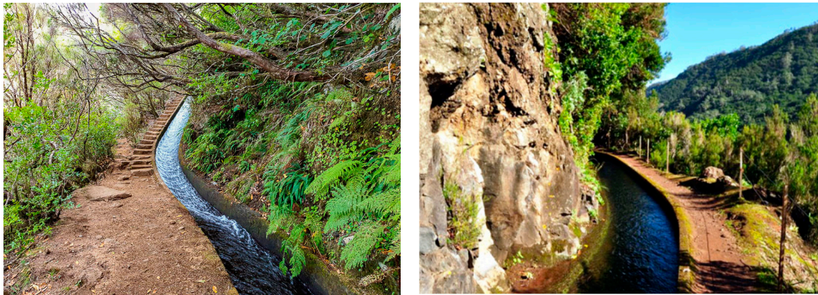
Figure 18. Levadas Canal on Madeira Island.
