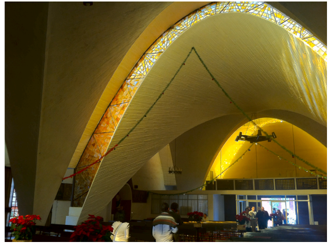
Fig. 3. “San Antonio de las Huertas” church in Mexico City. A succession of groined vaults with free edges. (Image: C. Lázaro).
