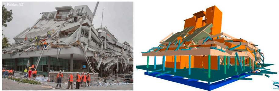
Fig. 7. Pyne Gould building collapse comparison between real (left) and simulated (right) collapse shape [64].
