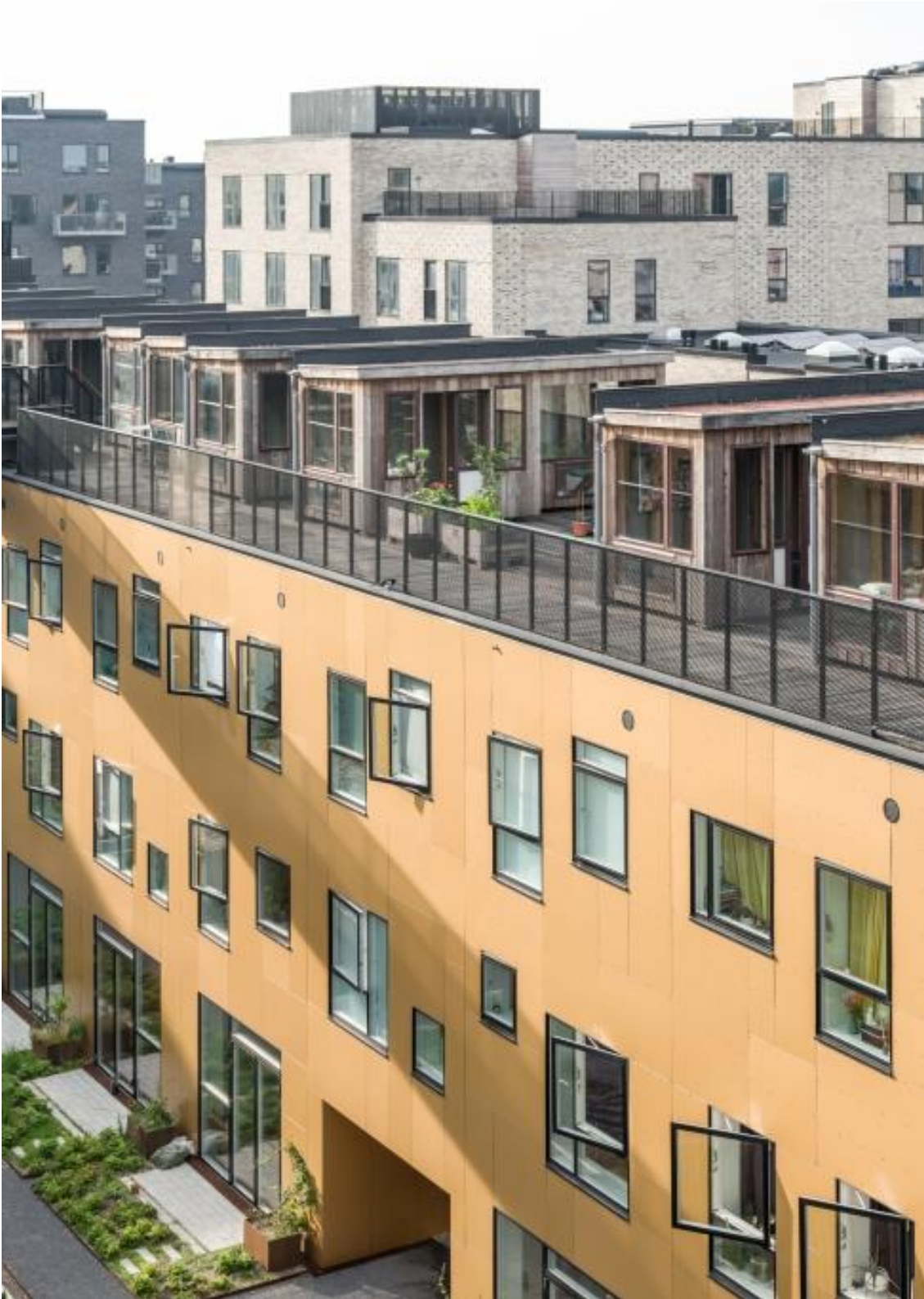
Fig. 58. Fachada en Patio interior (Lendager, 2020) Fuente: https://lendager.com/project/resource-rows/
