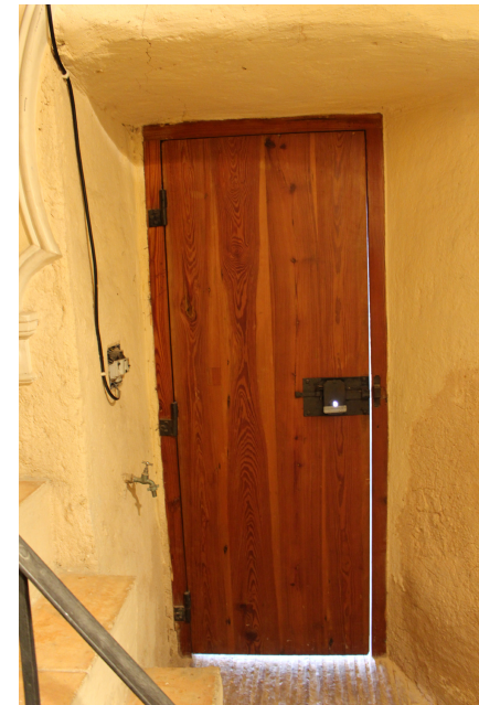
Interior puerta principal
