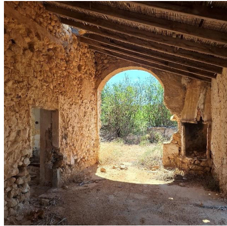
Figura 4. Romany, Casa Fornés, 2024
