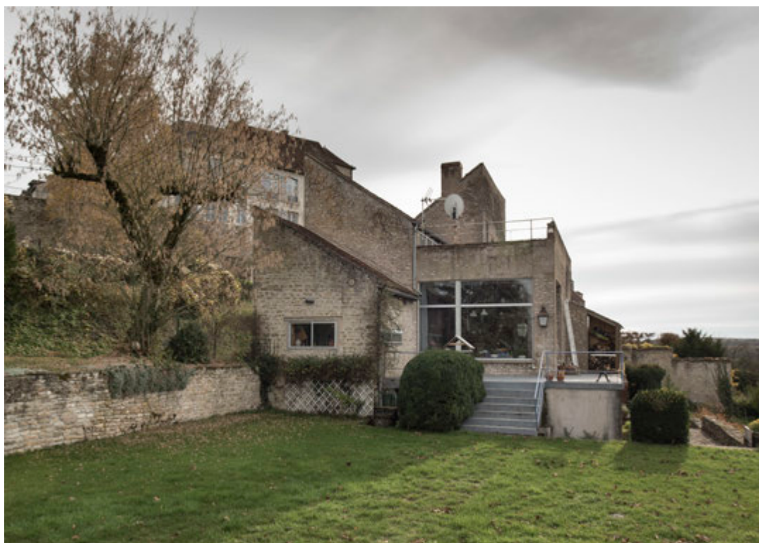
FIG. 43 Maison Renaudin-Battanchon from North, showing the kitchen extension on the left (Photo Tim Benton).
