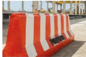
Muros New Jersey
