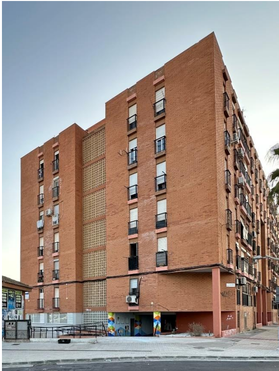
Figure 71. View of dwellings in Alfafar
