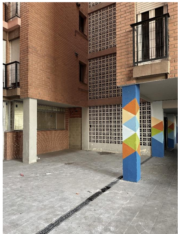
Figure 74. View of dwellings in Alfafar
