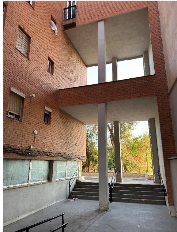
Figure 72. View of dwellings in Alfafar
