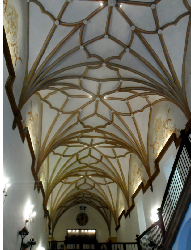
Fig. 18. Interior view of the restored vault. (Source: Own elaboration).
