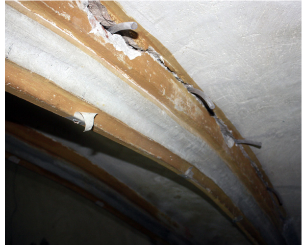
Fig. 12. Mortar injections and stitching with fiberglass rods. (Source: Own elaboration).
