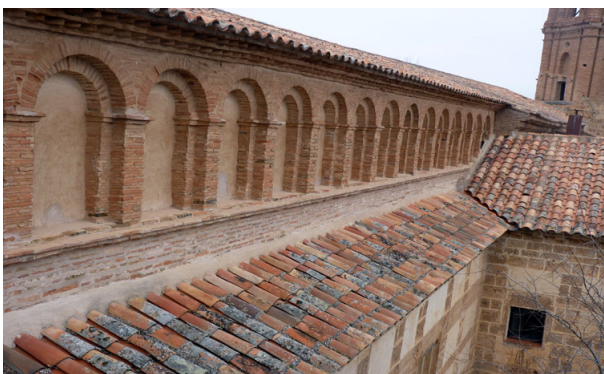
Fig. 15. Blocked gallery of small arches on the longitudinal façades. (Source: Own elaboration).
