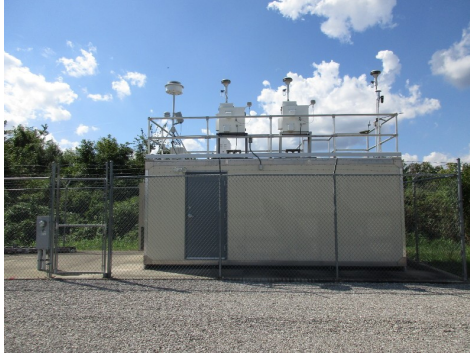
Figure 2.1: Example of an air quality monitoring station [34].
