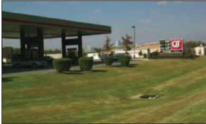
Figure 20.- Filter strip in a road area. (MDDEP and MAMROT, 2012)
