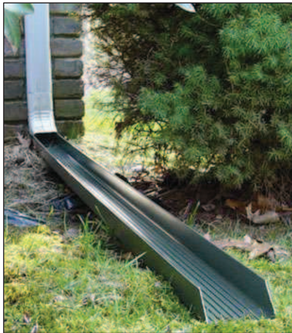
Figure 11.- Downspout disconnection. ( www.centurywaterproofing.com )
