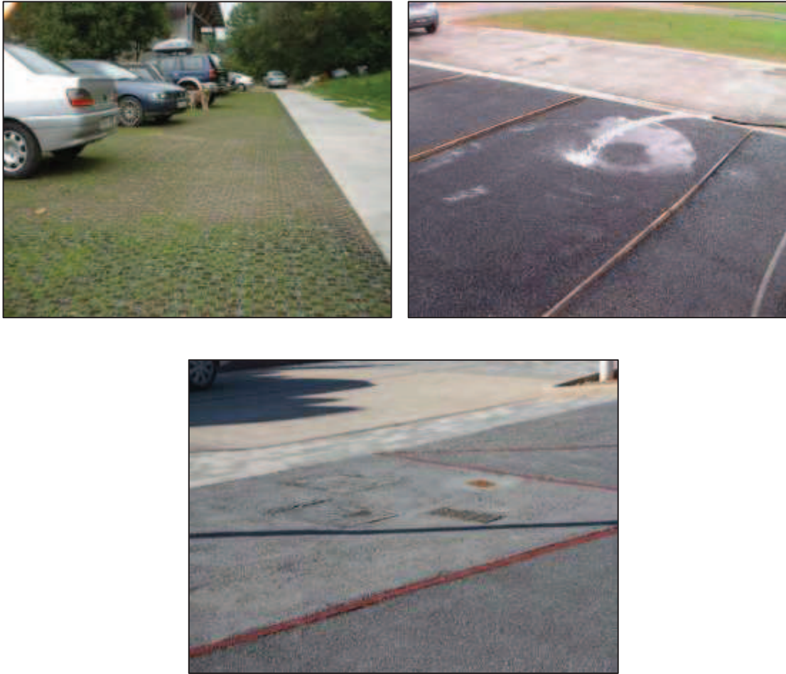
Figure 18 a,b,c.- Different types of porous pavements. From left to right and from top to bottom: plastic grid, porous asphalt and porous concrete (Sources: www.gitco.unican.es and Dr. Ignacio Andres Domenech).
