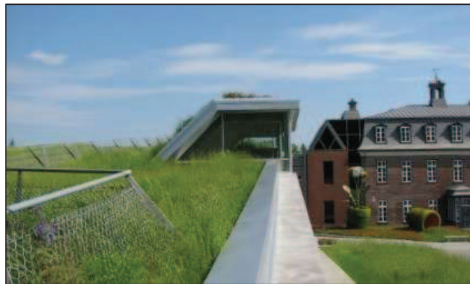
Figure 6.- Extensive green roof of the Charlesbourg Library, Quebec. ( www.trait-carre.org )
