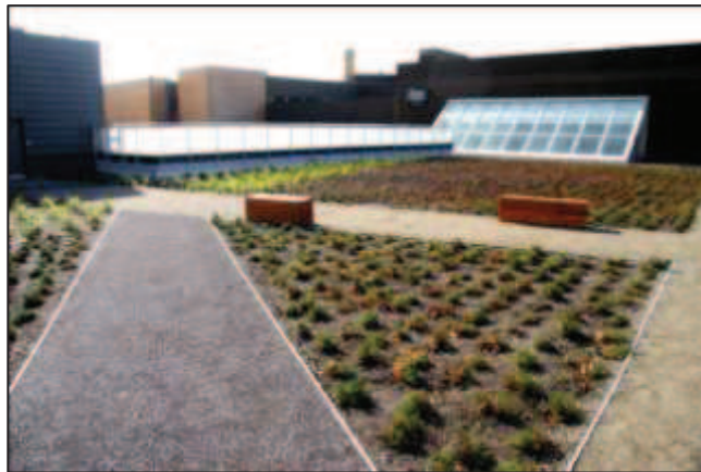
Figure 5.- Intensive green roof in the CEGEP of Limoilou, Quebec. ( www.climoilou.qc.ca )
