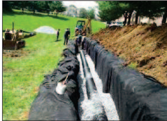
Figure 13.- Infiltration trench under construction. (TRC and CVC, 2010)
