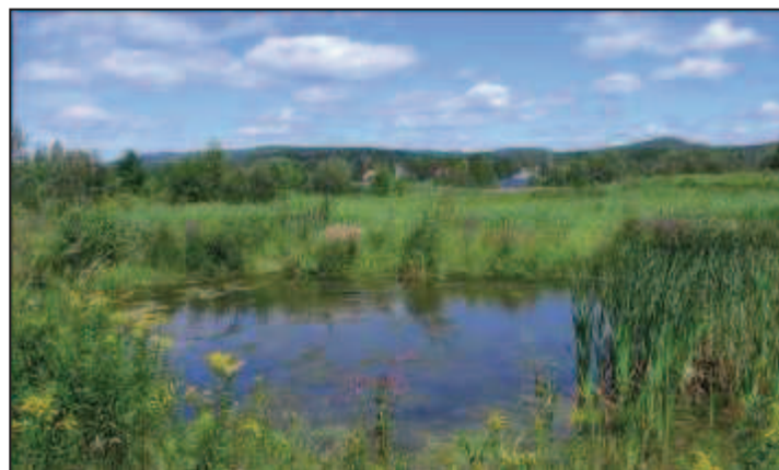
Figure 33.- Constructed wetland in Quebec. (MAMROT, 2010)
