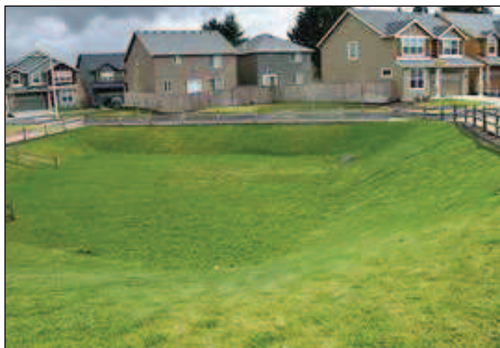
Figure 29.- Detention basin in a residential area. ( www.stormwaterpartners.com )
