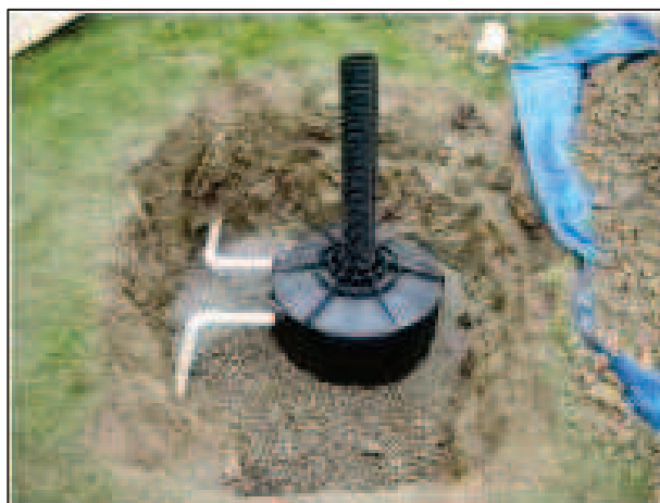
Figure 14.- Dry well under construction. (www.agry.purdue.edu)
