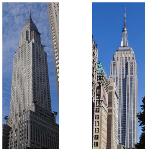
Imagen 3. Chrysler Building y Empire State Building, New York
