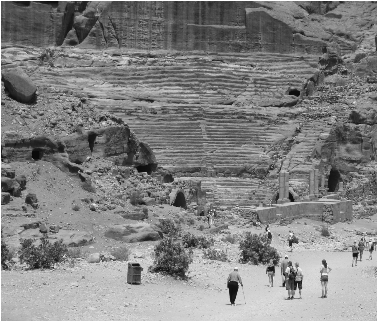
Figure. 5. The Petra Theatre: between the task of ATHENA IRP team there is the one of defining “guidelines for compatible utilization” and “Ancient theatre usage manual” for the network of ancient theatres belonging to the partnership and characterized by different problems and opportunities (Photo: Francisco Juan Vidal)
