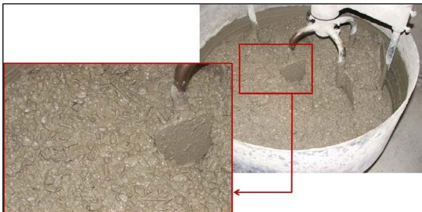
Figure 7. Concrete mixing: a detail.
