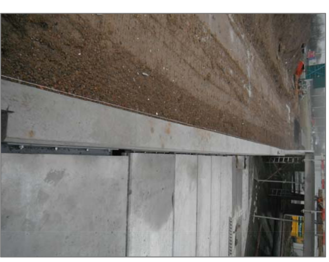
PLACEMENT RAMP PLATES
