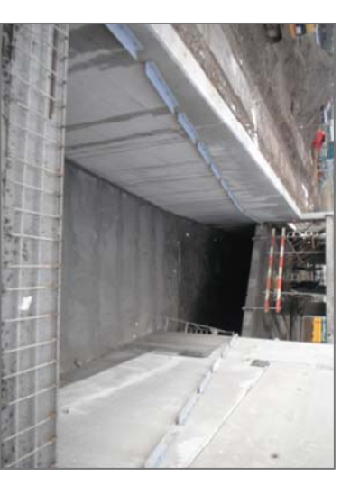
METALLIC SUPPORTS FOR THE RAMP PLATES
