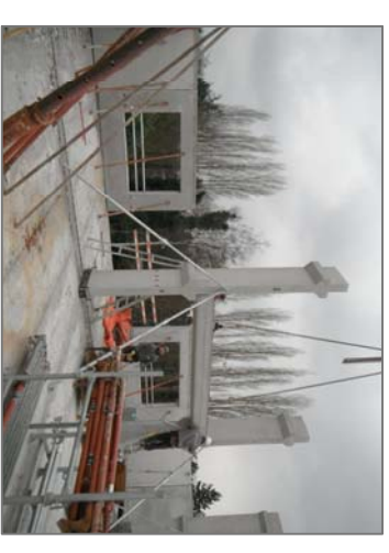
PLACEMENT PREFABRICATED COLUMNS
