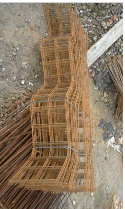
Placement of separators, to separate the upper and lower reinforcements.
