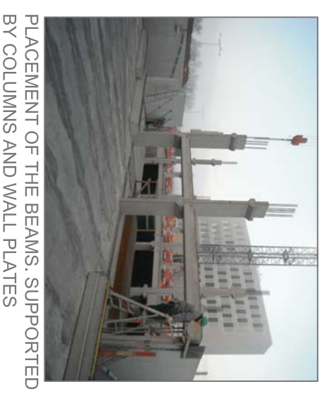
PLACEMENT PREFABRICATED BEAMS WITH SPECIAL CRANE HOLDER
