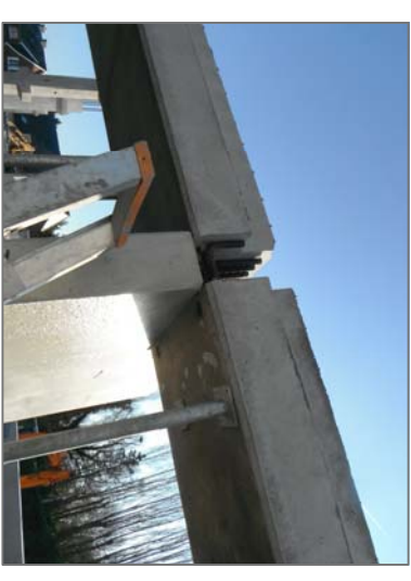
JOINT COLUMN-BEAM
