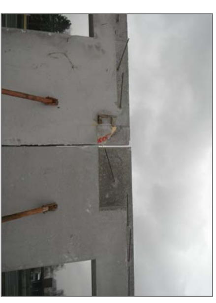
CONNECTORS FOR THE BEAMS AND FLOOR PLATES IN THE WALL PLATES
