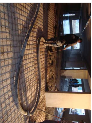
PLACEMENT OF THE STEEL MESH
