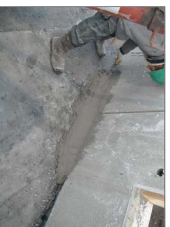
CONCRETING JOINTS TO SECURE THE LINK
