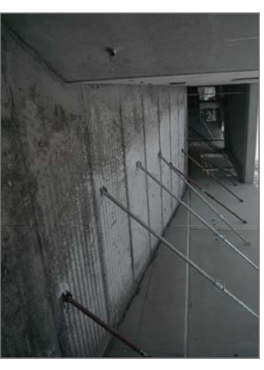
WALL PLATES SUPPORTED BY SCHAFFOLDINGS
