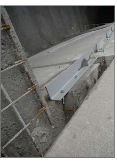
METALLIC SUPPORTS FOR THE RAMP PLATES
