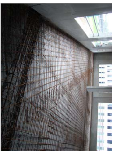
PLACEMENT OF THE STEEL MESH
