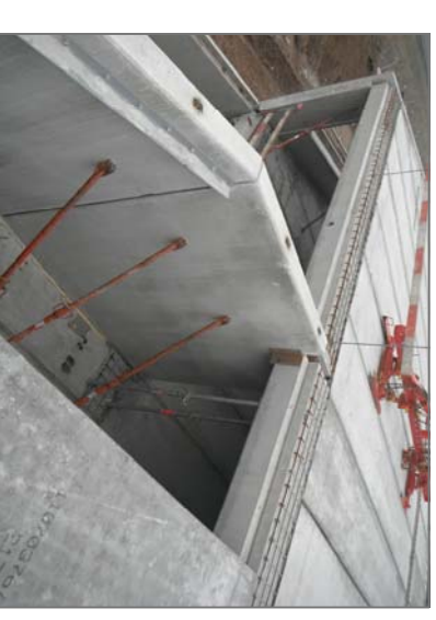
FLOOR PLATES. PLACEMENT WITH SPECIAL CRANE HOLDER
