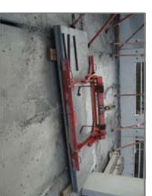
SPECIAL GRABS FOR THE PLACEMENT
