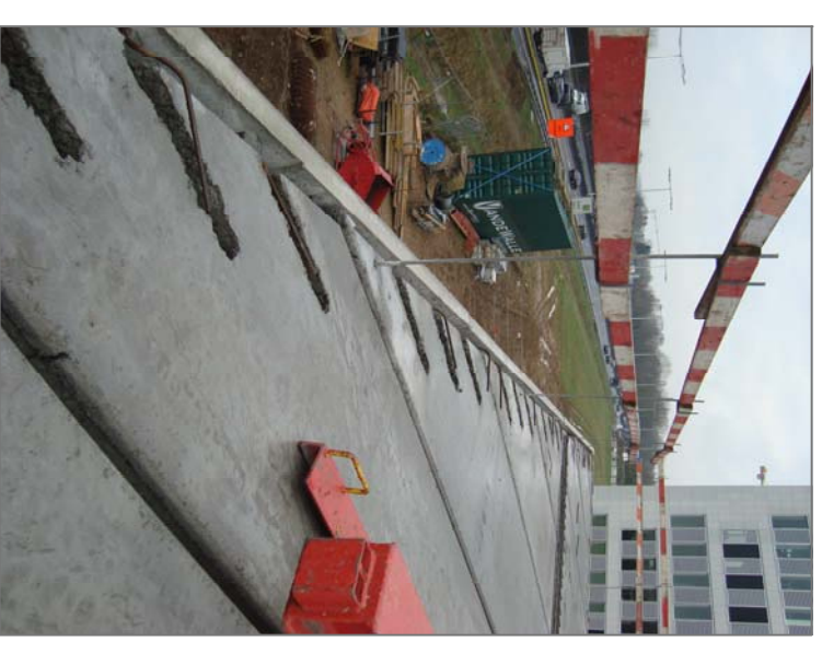
CONNECTORS REINFORCEMENTS TO LINK THE STRUCTURE
