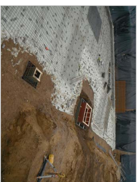
Placement of the lower reinforcement of the foundation slab.
