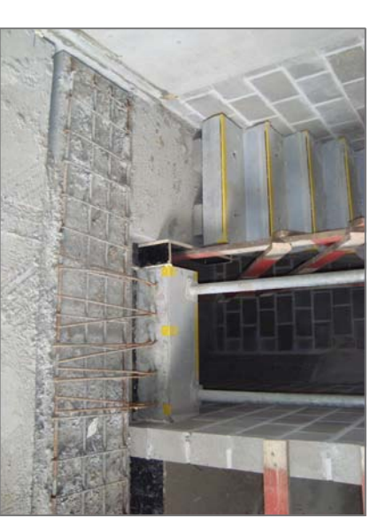
CONNECTORS REINFORCEMENTS WITH THE BEAMS
