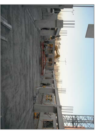
PLACEMENT PREFABRICATED BEAMS WITH SPECIAL CRANE HOLDER
