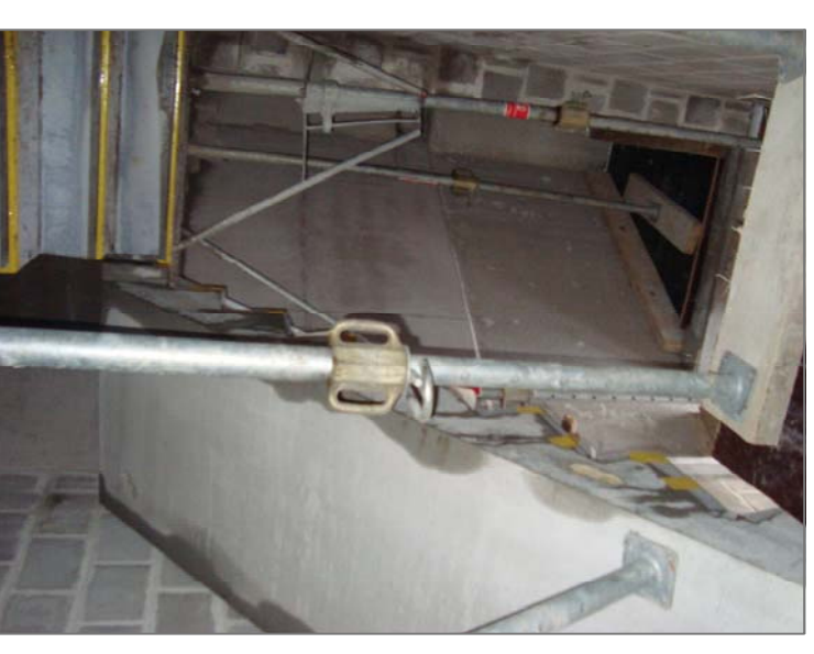
PREFABRICATED STAIR SLAB SUPPORTED BY SCHAFFOLDINGS
