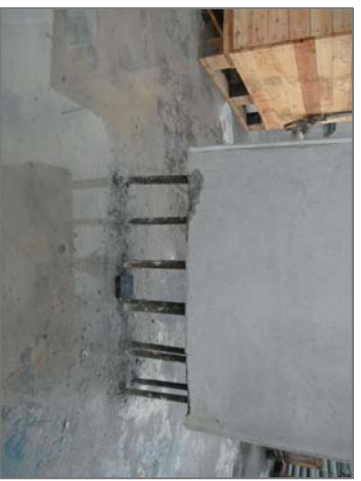
COLUMNS STEEL CONNECTORS
