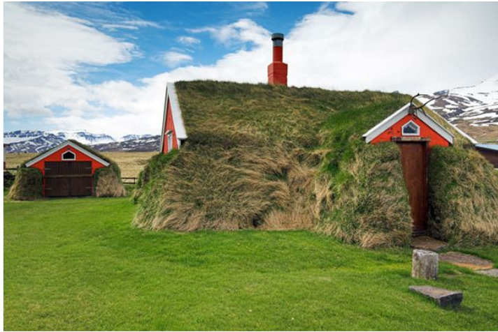
Turf house in Bakkagerdi, north east Iceland. This is a traditional style of house building in Iceland, offering superb insulation from the harsh environment.
