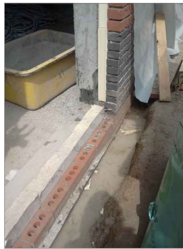
DETAIL 2: FACADE STARTING-WINDOW S:1/10
