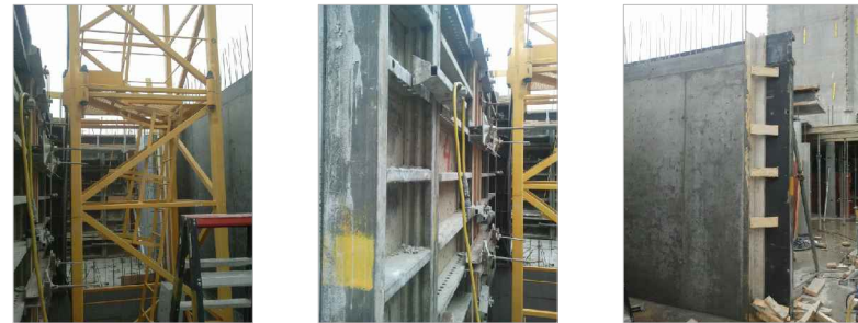
STEP 33: FORMWORK WALLS _ S:1/40
