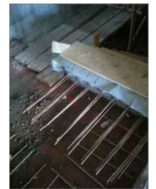
DETAIL 11.2: UNION PREFABRICATED STAIR-IN SITU FLOOR _S:1/10
