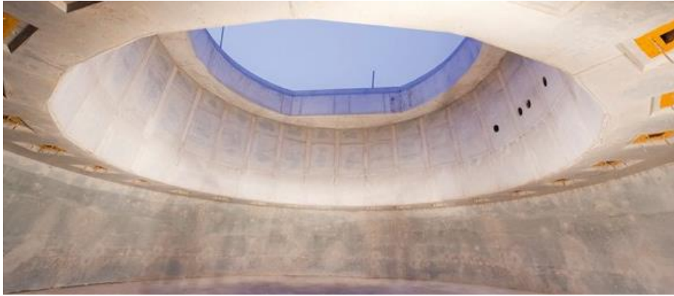
The final foundation
