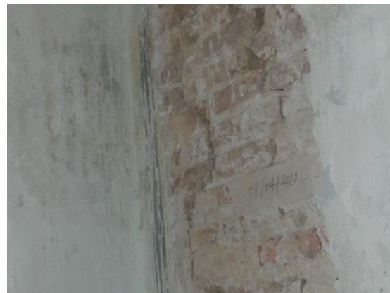
Picture 143. Plaster test for the crack's state check
