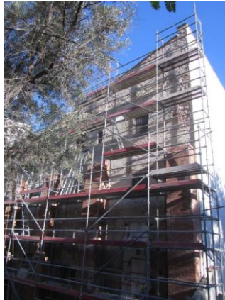
Picture 138. Scaffolding on West façade (48)
