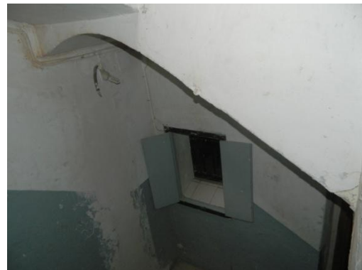
Graphic 38. Brick up vault's outline and construction (33)
