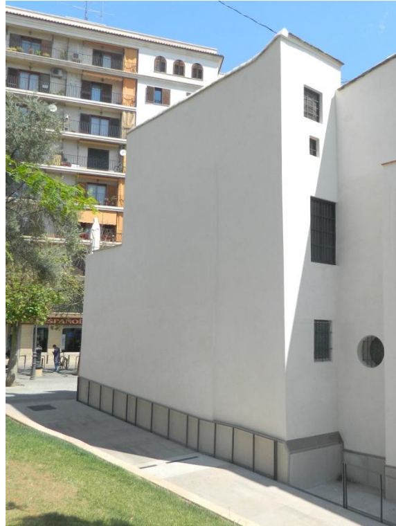
Picture 38. West Façade's left side view
