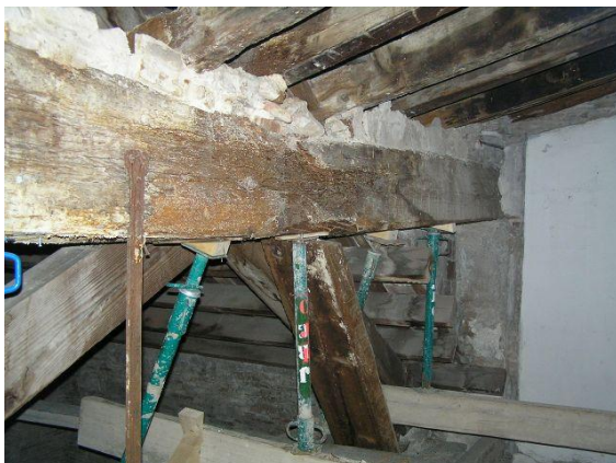
Picture 134. Former wood beam struted (44)
