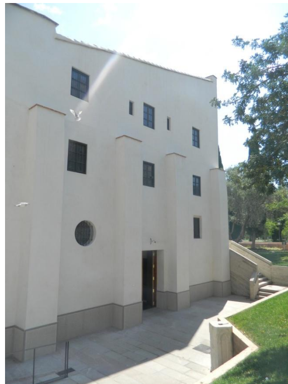
Picture 40. West Façade's right side view
