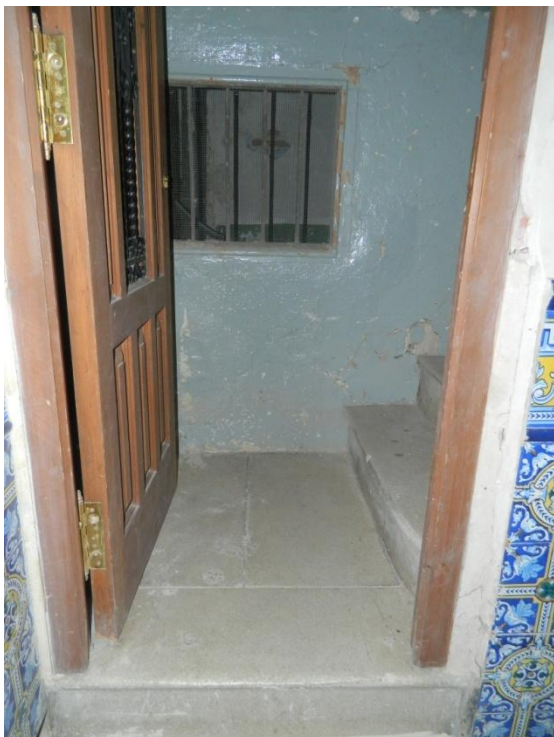
Picture 57 Access to the stairs
