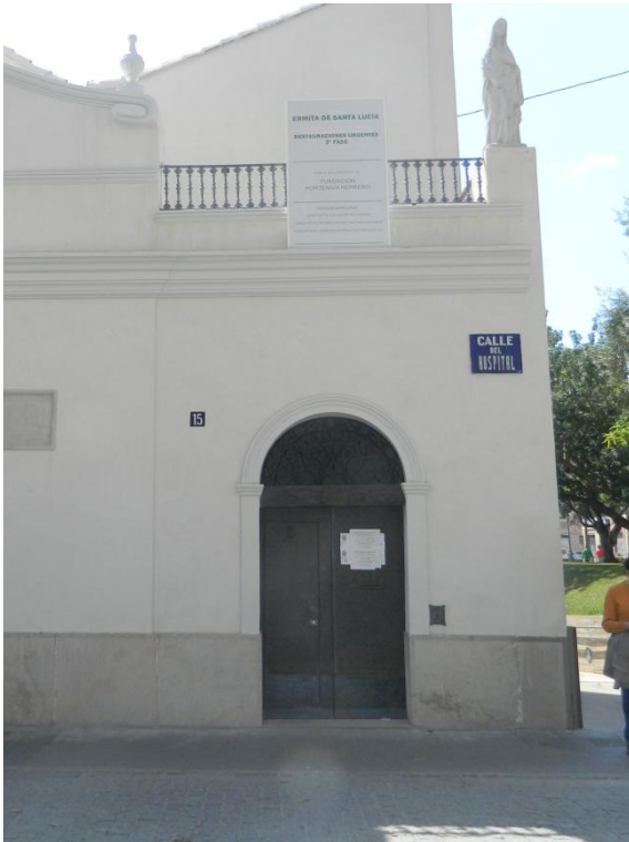
Picture 30. Hermitage access at the North Façade
