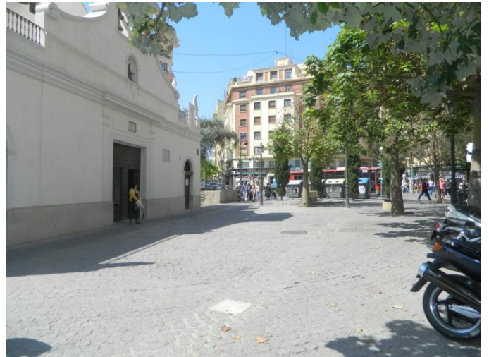
Picture 21. North Façade access by the square
