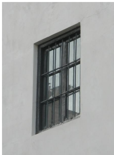
Picture 145. Exterior window sight
