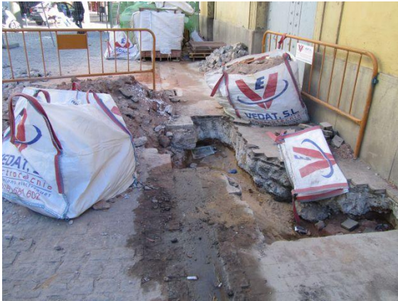
Picture 136. Street excavation (46)
