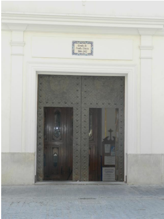
Picture 26. Main door in the North Façade
