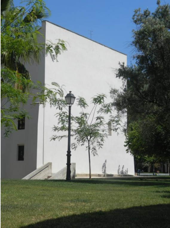
Picture 41. South Façade's corner with the West Façade
