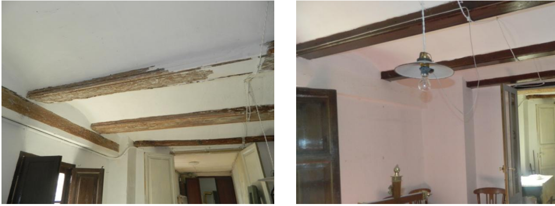
Pictures 104 and 105. Interior vault floor structures (18th and 19th Centuries respectively)
