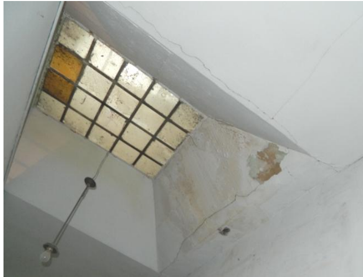
Picture 149. Skylight over the first floor corridors
