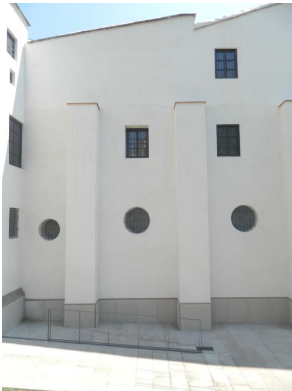
Picture 39. West Façade's central part view
