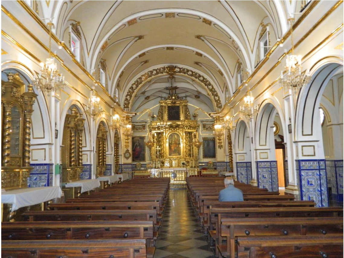
Picture 47. Principal nave's frontal view, with the barrel vault on the top and the Gothic vault at the end
