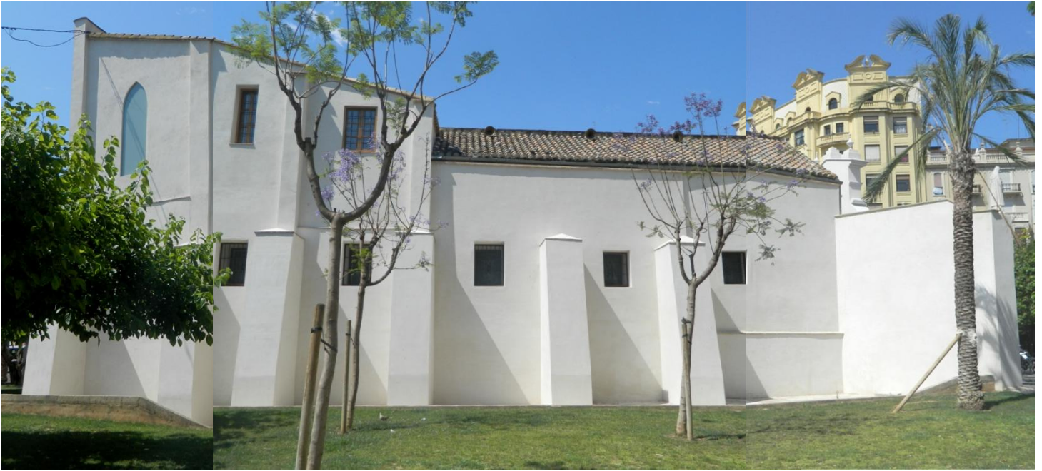
Picture 45. East Façade frontal view
