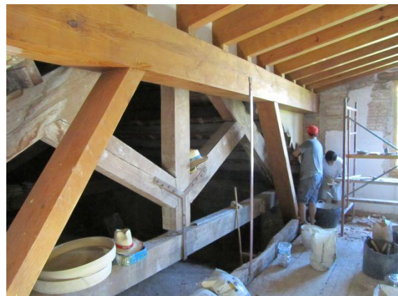
Picture 135. New wood beam (45)
