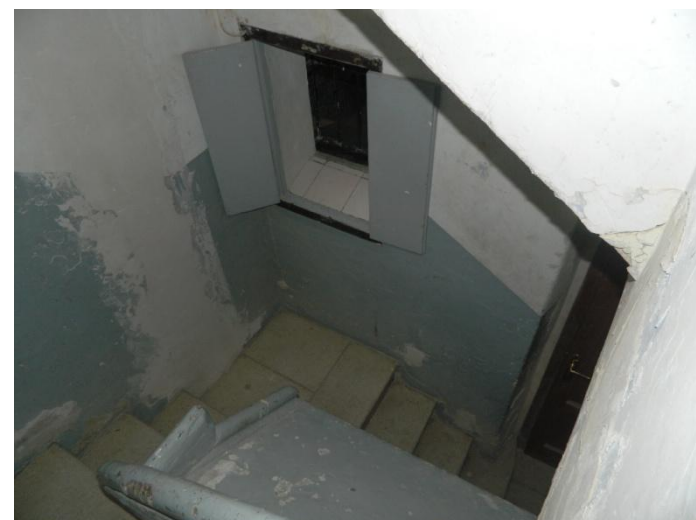
Picture 58. Stairs to access to the first floor
