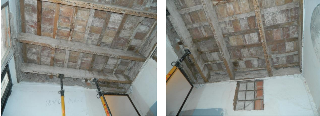
Picture 157 and 158. Different views from the floor structure.
