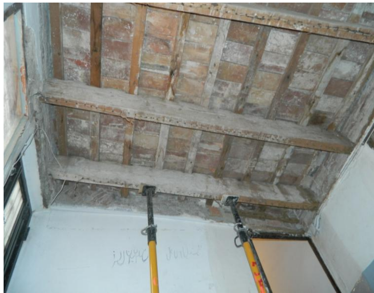
Picture 147. Wood beam strutted
