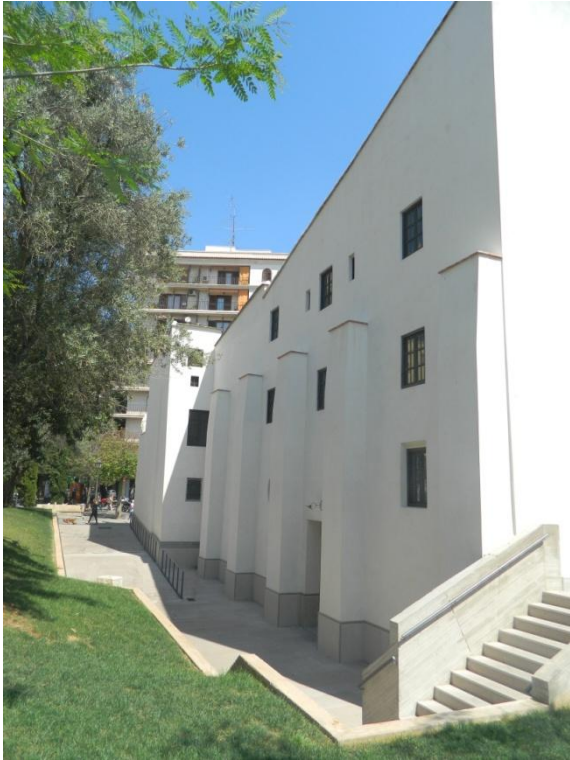
Picture 37. West Façade view with the lateral corridor and the stairs to the South Façade
