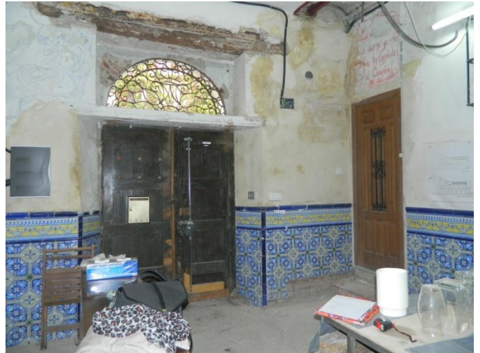
Picture 55. Brotherhood House Entrance Room from the North Façade
