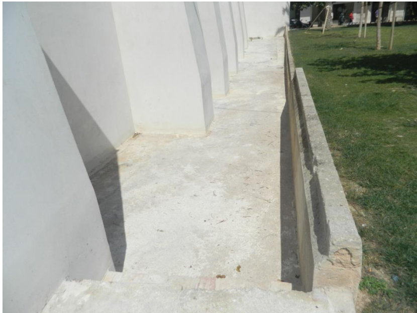
Picture 46. East Façade's lateral corridor
