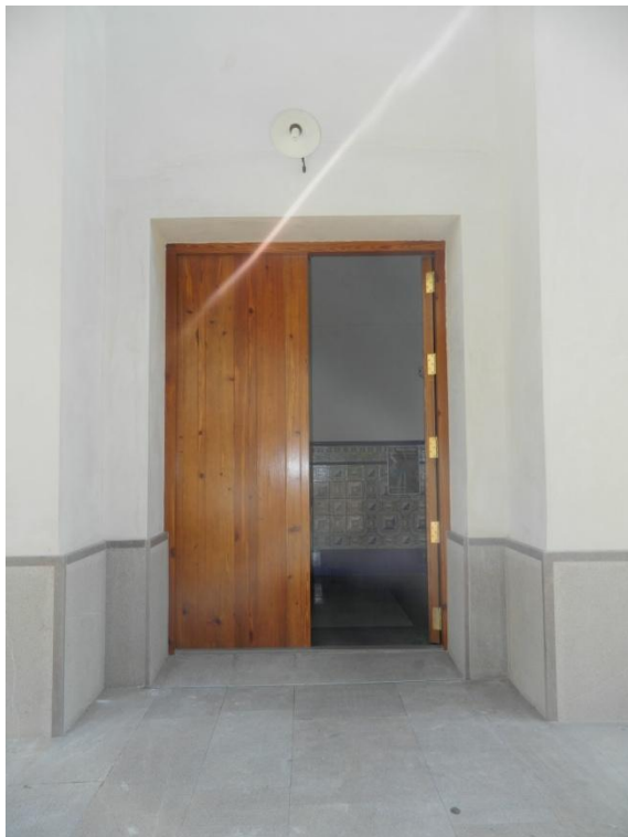
Picture 28. Door in the West Façade. Accessible entrance
