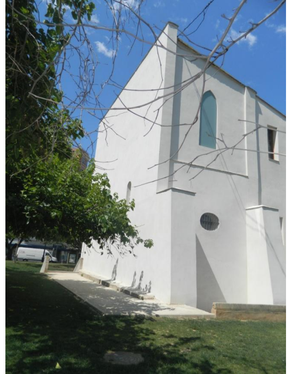
Picture 42. South Façade's corner with the East Façade
