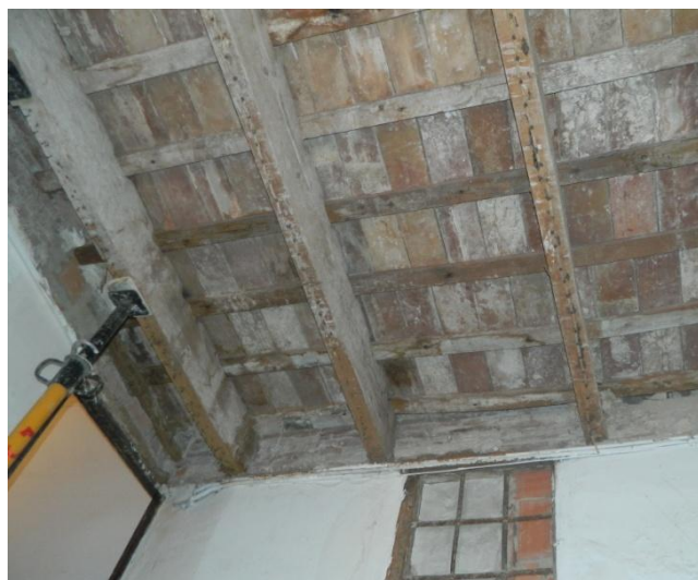
Picture 148. Wood beams fixed into the brick wall
