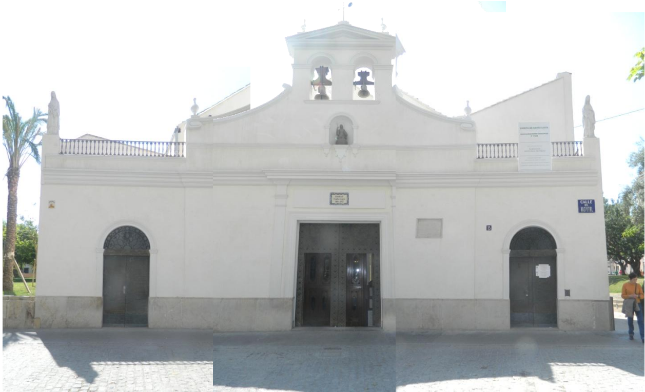
Picture 34. North Façade frontal view
