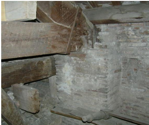
Picture 116. Wood truss resting over a pillar (35)
