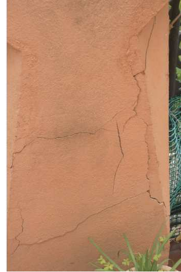
Cara Interior pilastra
