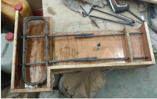
Figure 5.32: Formwork of the elements
