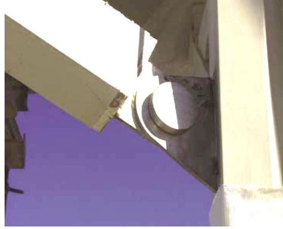
Figure 2.52: Detail of the steel bolted connection
