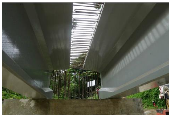
Figure 2.47: Transversal connection between the T beams
