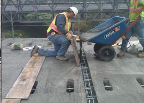
Figure 2.45: Filling the joints with UHPFRC
