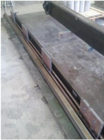
Figure 5.65: Mould of the bottom chord before pour the concrete
