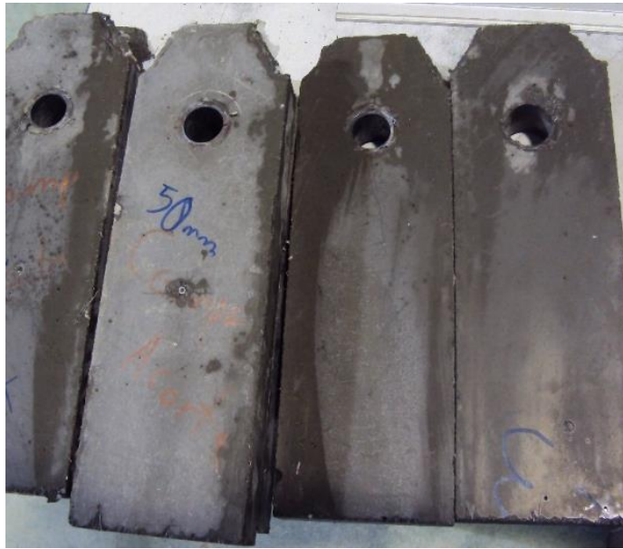
Figure 5.79: Compressive diagonals after sewing
