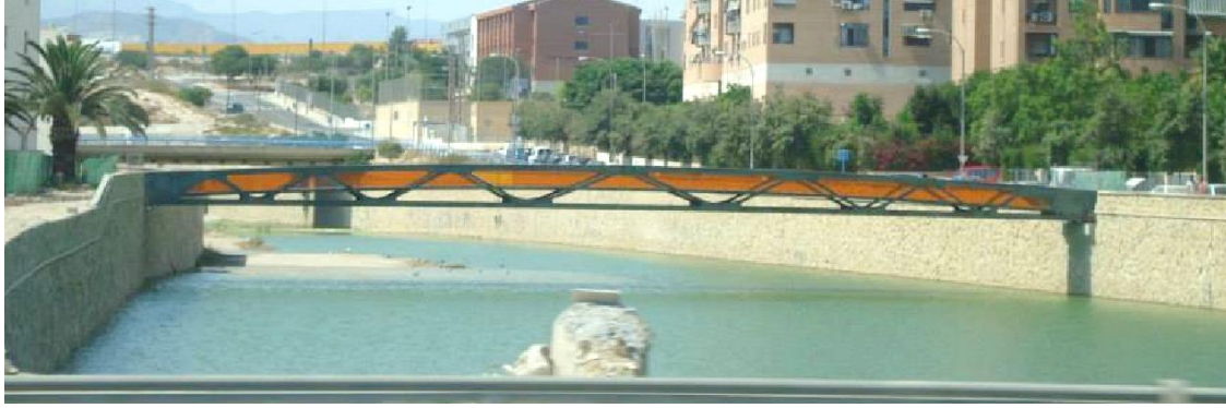
45 m span truss footbridge at Alicante. UPV group
