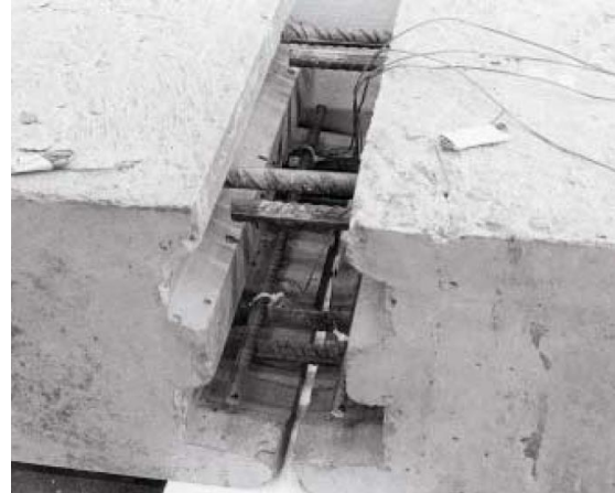
Figure 2.50: Connection between CRC elements
