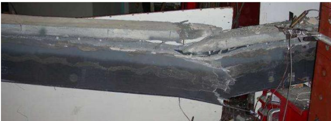
Figure 2.60: Failure of the tested beam
