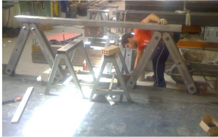
Figure 5.66: Truss during the assembly process
