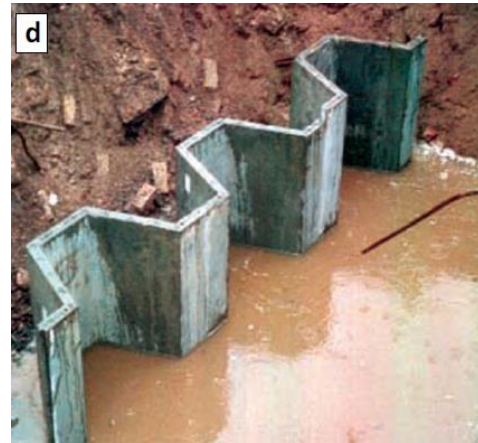
Figure 3.38: Sheet piles already placed
