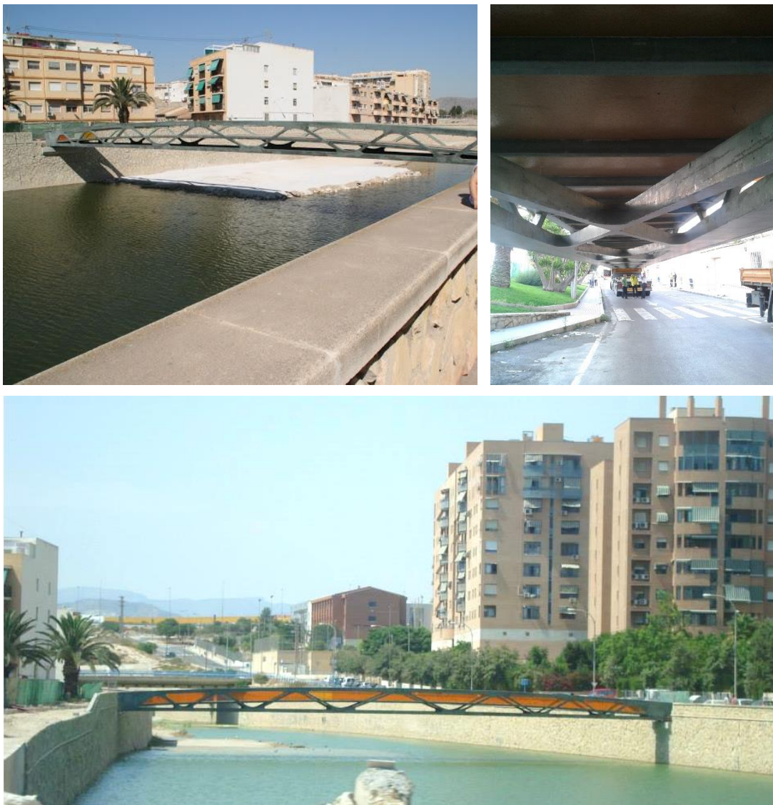
Figure A.14: Bottom view of the footbridge during the placing and final view
