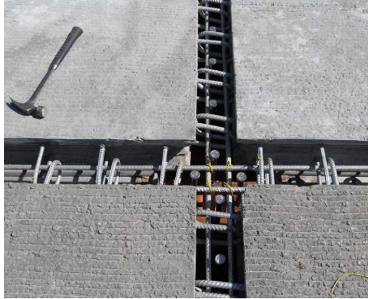
Figure 2.44: Intersection of the center line joint and transverse joint prior to filling
