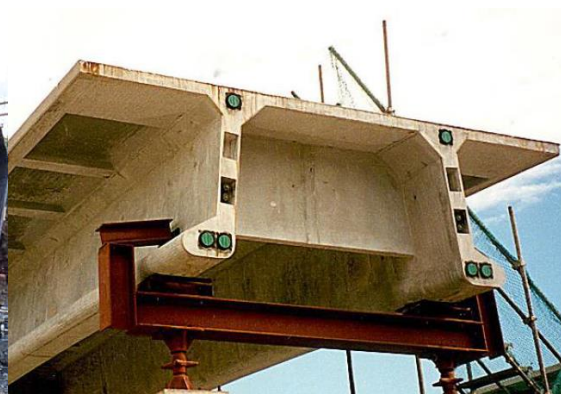
Figure 2.40: Sakata Mirai footbridge in the construction process
