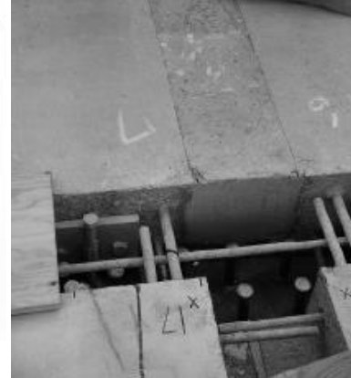
Figure 2.42: One of the joints of the CN Ride Overhead Bridge
