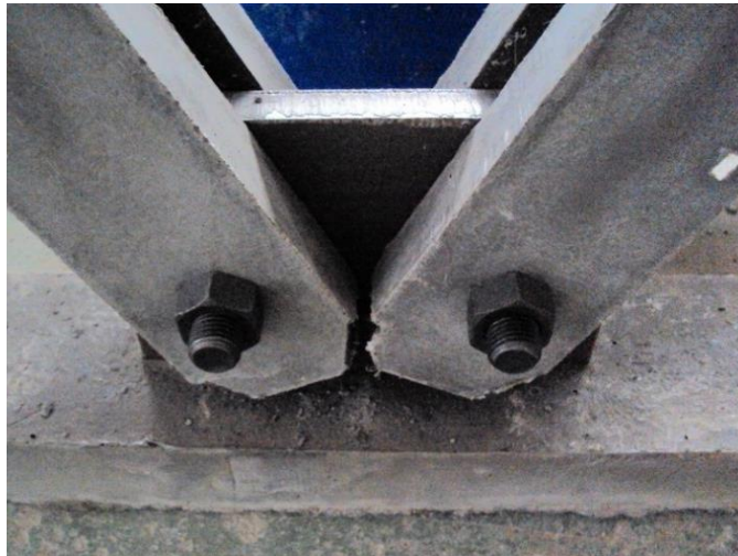
Figure 5.68: Detail of the bottom chord connection
