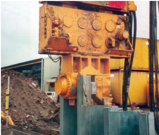
Figure 2.37: UHPFRC sheet piles being hammered
