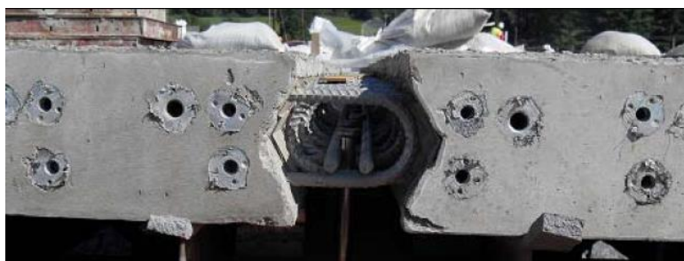
Figure 2.43: Detail of the connection between two panels
