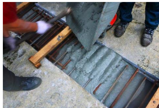
Figure 2.48: In-situ concrete being poured
