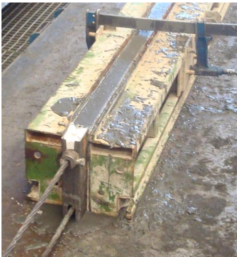
Figure A.5: Tie being cast at the precast company
