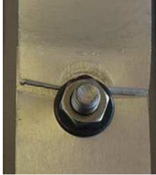
Figure 5.8: Failure on steel plate
