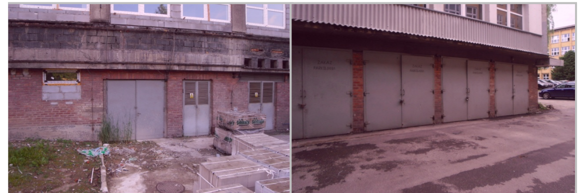
Photography 26. North elevation.
