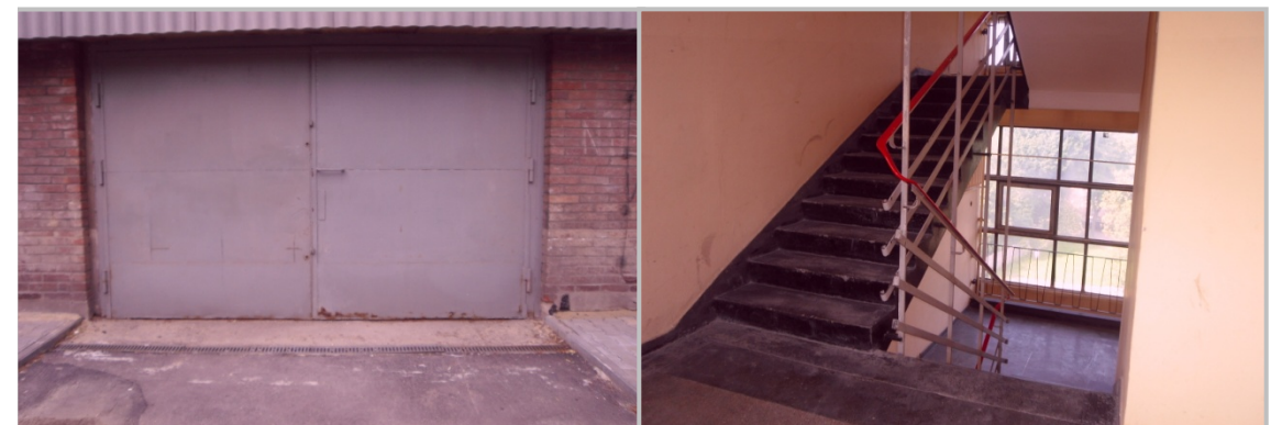
Photography 28. North elevation
