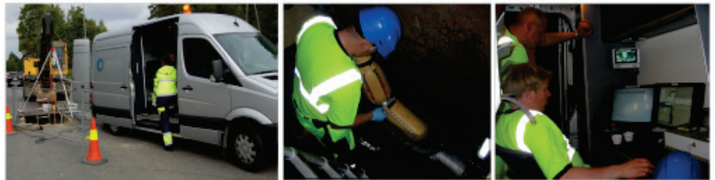
Figure 2.2. The inspection unit and PipeScanner field operation
