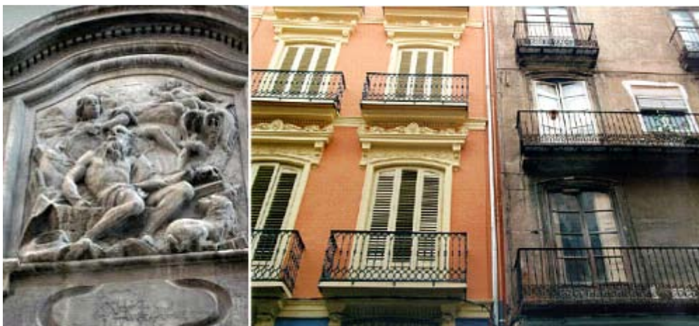
Figure 4. Works done in the Velluters neighborhood areas of intervention
