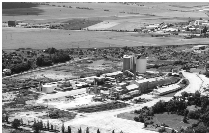
Fig. 1. Industrial plant location
