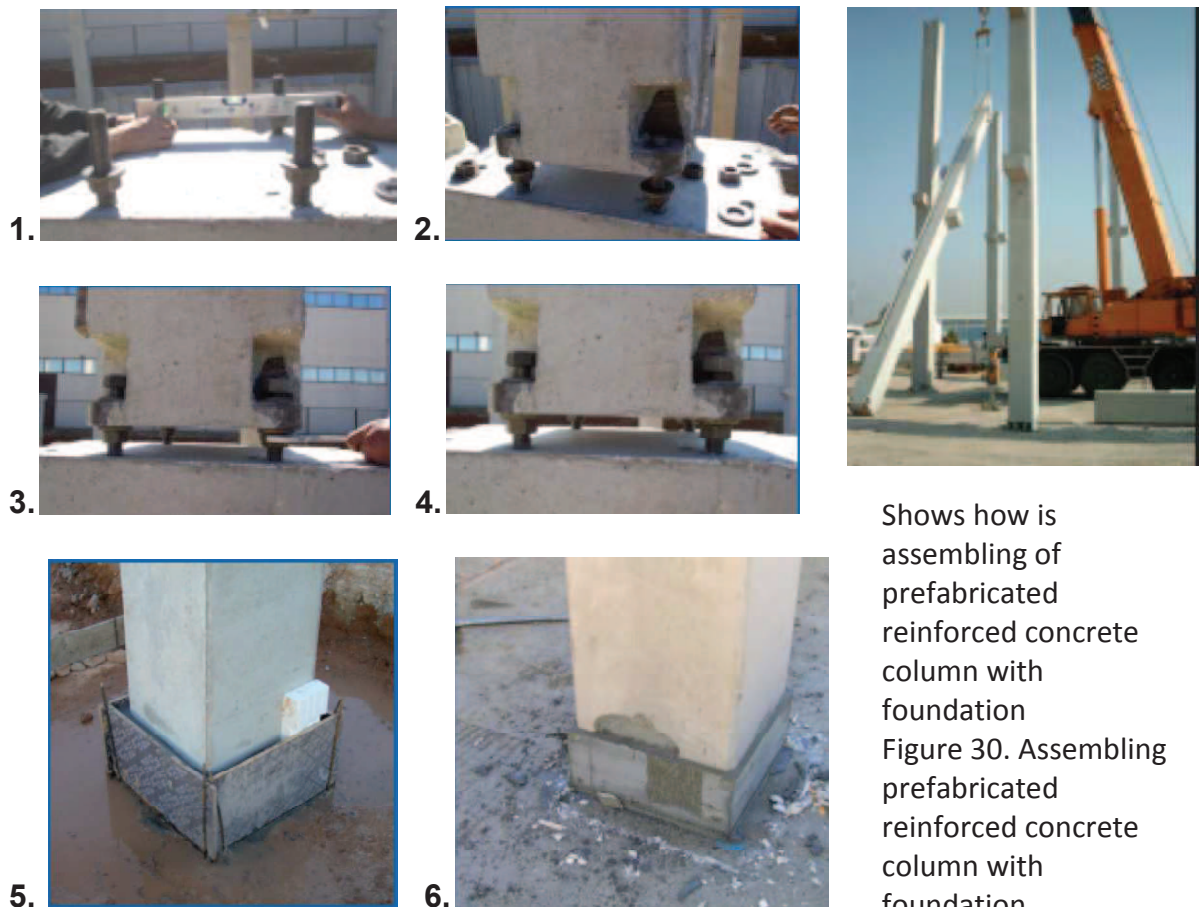
Figure 30. Assembling of prefabricated column
