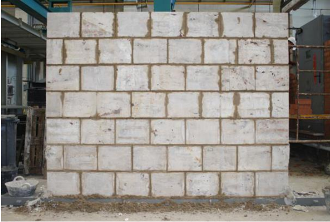
Figure 1. Ashlar inhomogeneous masonry wall.
