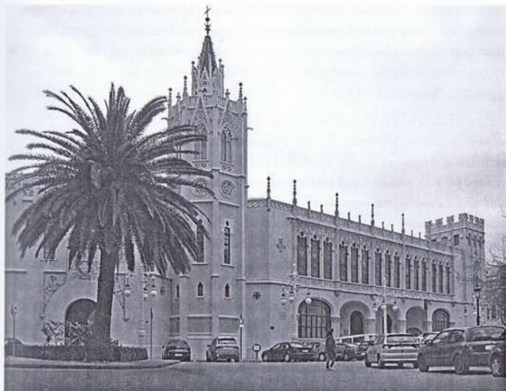
Figure 4. Municipal Pavilion of the Expo, Valencia, 1909. The Municipal Pavilion of the Expo was the result of interpretation and amalgam and a sample of local religious and civil gothic architecture, and was a token of similar interpretations of local tradition built both in the city and for other world's fairs. (Fernando Vegas and Camilla Mileto)
