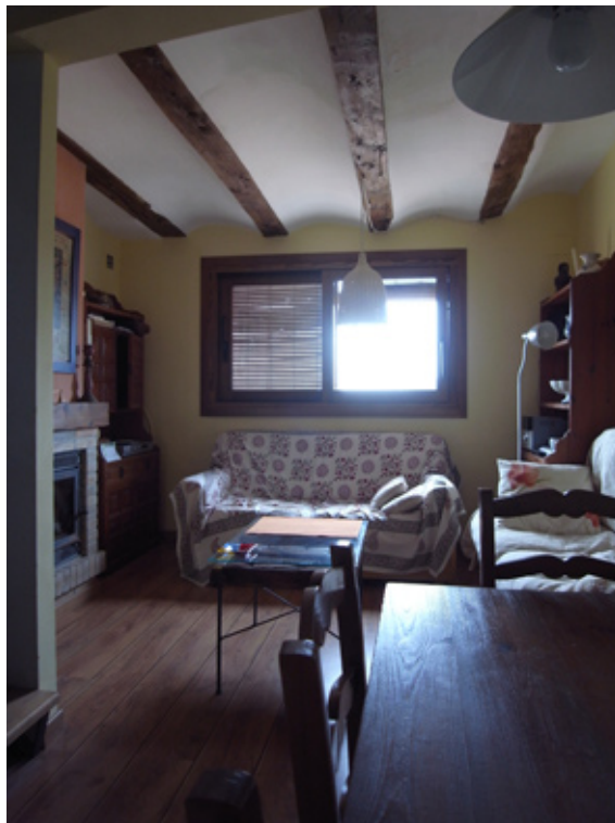
Photo2.6 Jack arch floor
