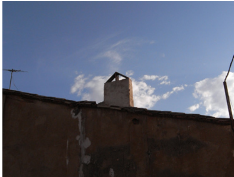
Photo1.4 The cover onto the short-edge of the chimney
