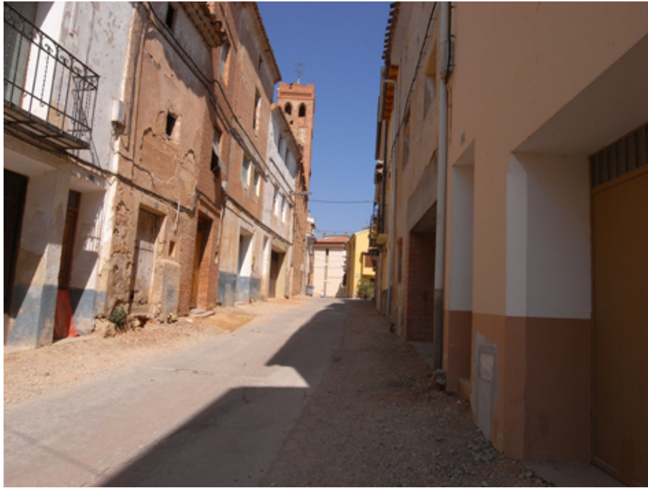
Photo3.1 Long line-unit in Torre Baja
