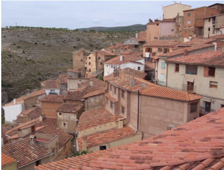
Photo3.5 Line-unit in Castielfabib
