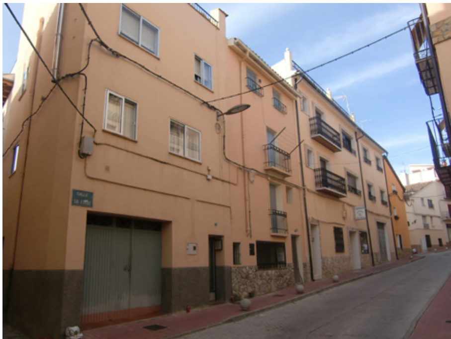
Photo3.2 Short line-unit in Torre Baja
