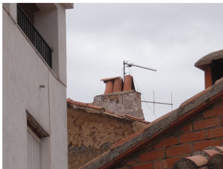
Photo1.5 The cover onto the long-edge of the chimney
