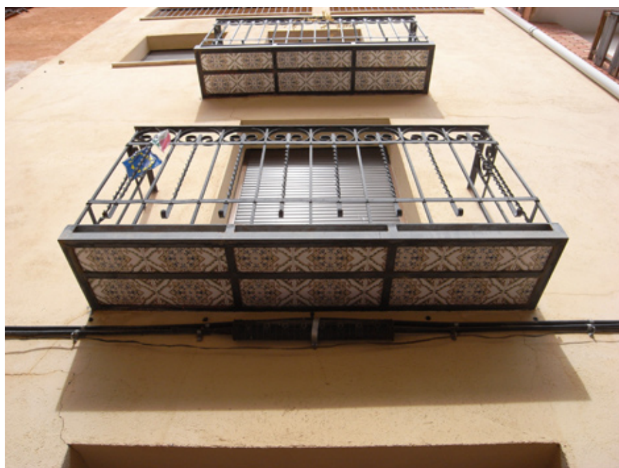
Photo4.2 The reverse side of the balcony is decorated with ceramic tiles.
