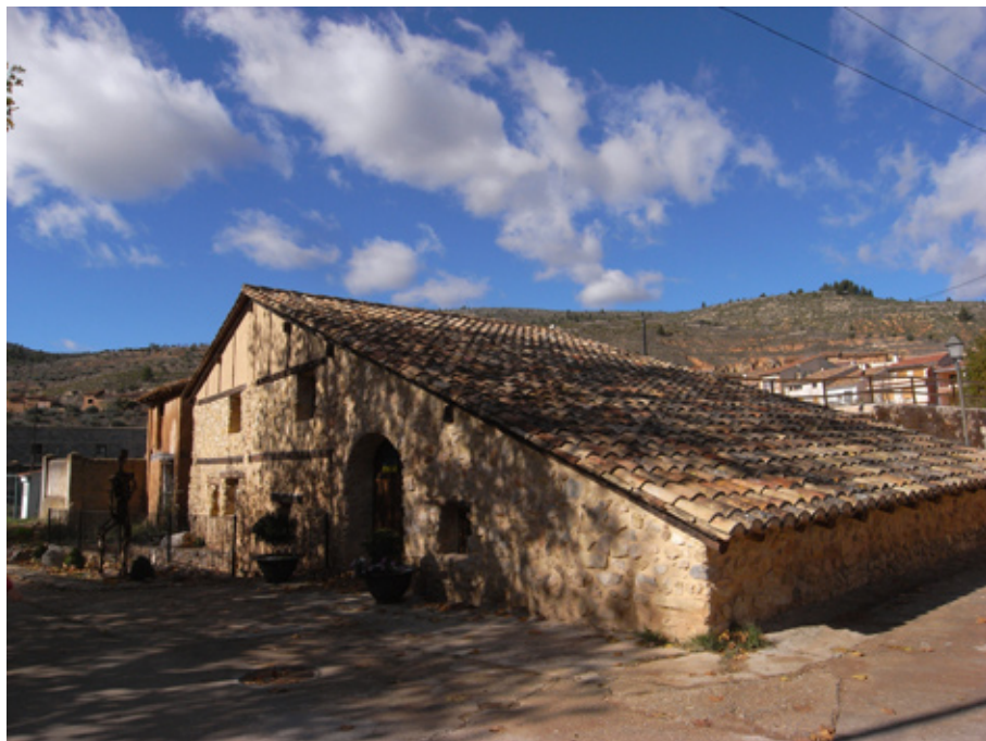
Photo3.17 The water mill in Casas Bajas
