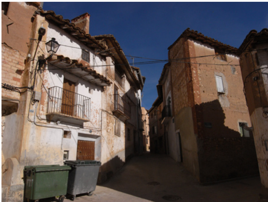
Photo3.4 Short line-unit in Casas Bajas
