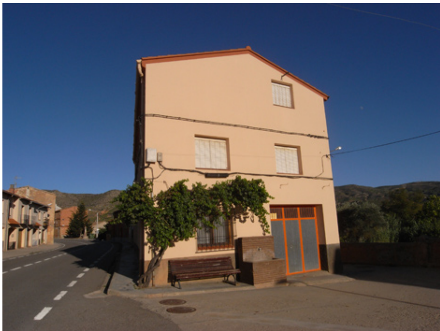
Photo3.18 The fountain point in Torrebaja
