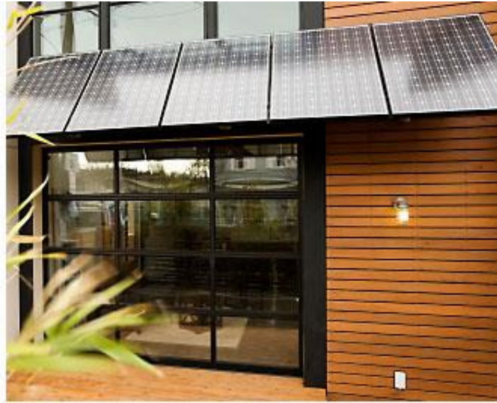
Figure 5. Shade mounted photovoltaic panels. ( http://www.solar-installation-pros.com/solar-carport.php )
