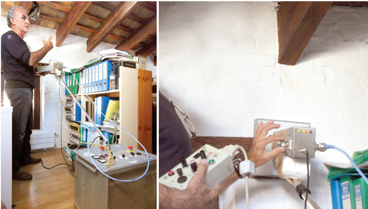
Fig. 7. Application of the microwave treatment on a timber lintel
