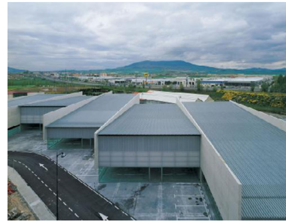
_ Office Silo Container Valle Iranguren
